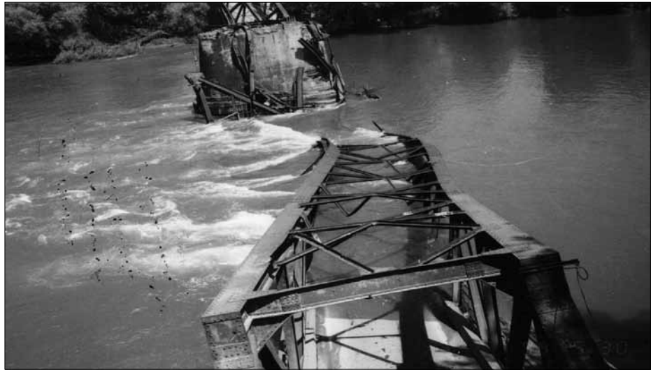
On 30 May 1999 already at the first run-up of two NATO fighter bombers F 16 the bridge of Varvarin was completely destroyed. The second run-up cost the lives of 10 people leaving 27 people seriously injured. (picture ma)
